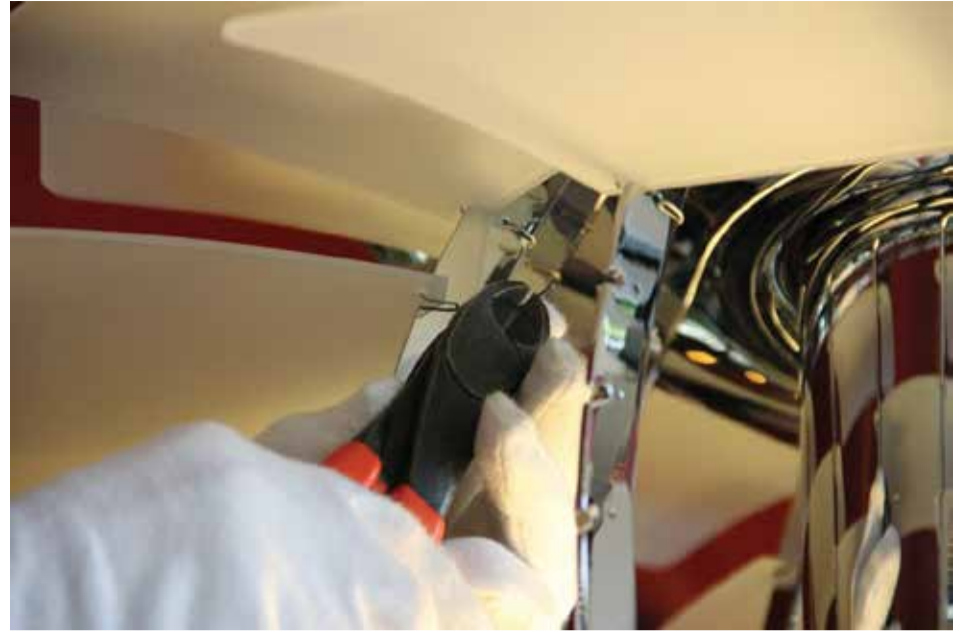
Figure 1.7 Trim wire to approximately 10mm and fold into leg pinch with pliers.
